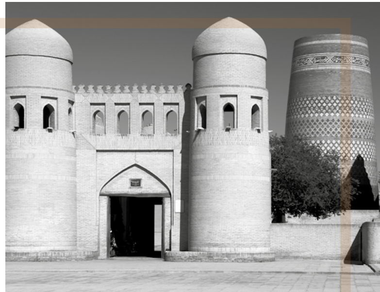
Western gate of the old part of the city of Khiva, Uzbekistan
