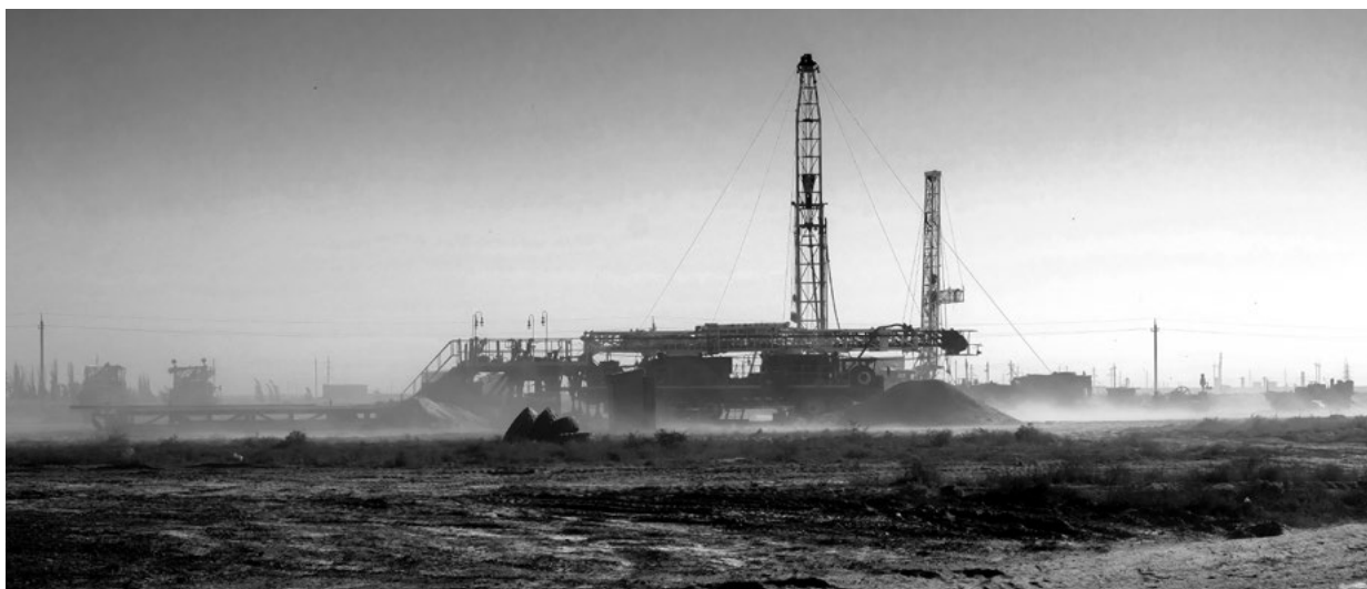
Drilling near Betpakdala, Kazakhstan
