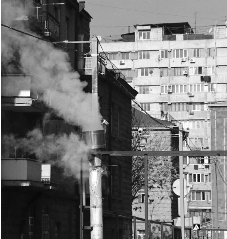
Heating system, Yerevan
