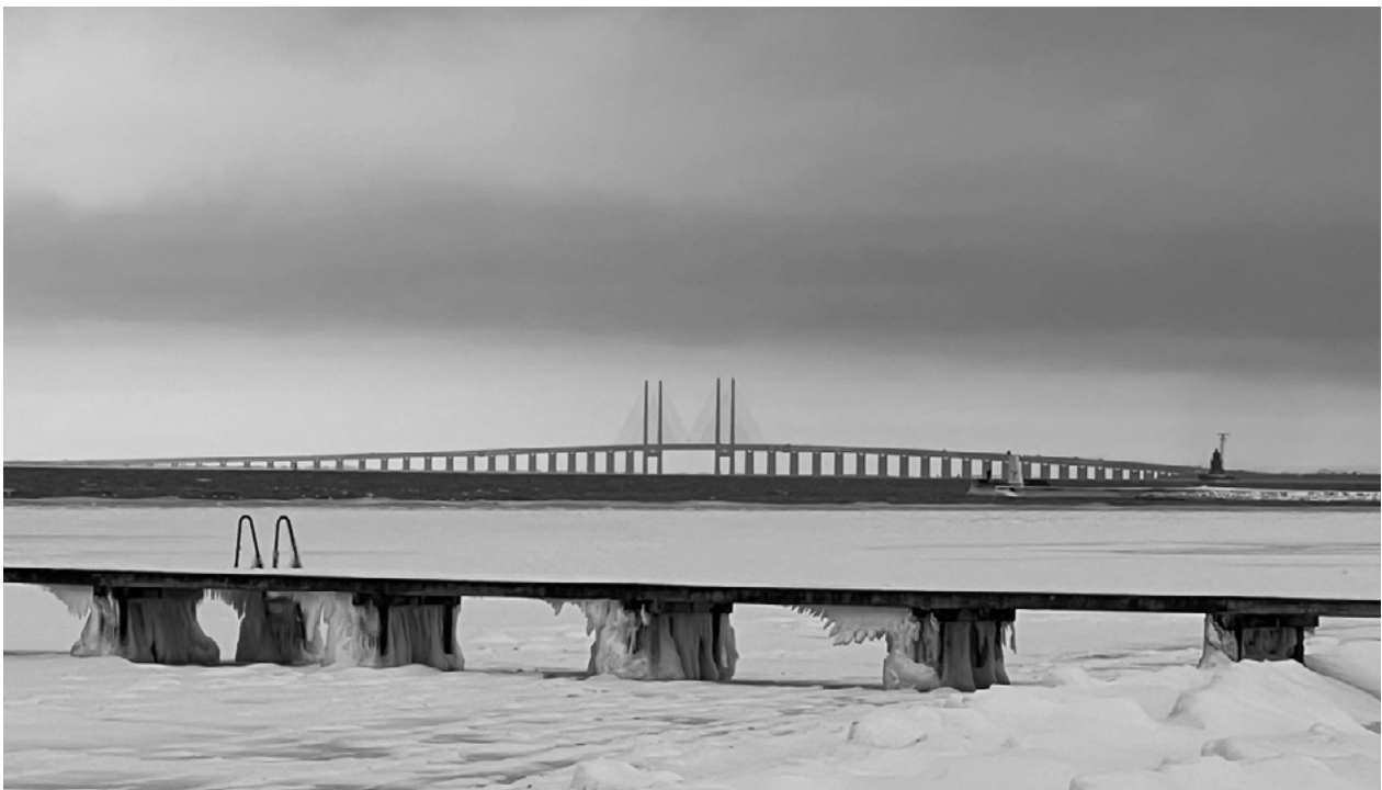
Bridge over Oresund
